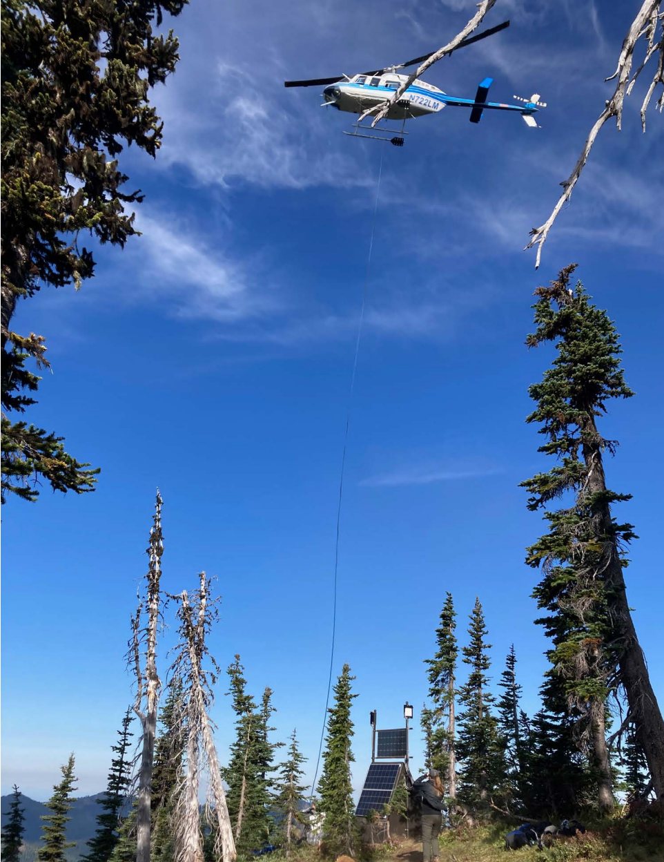
Photograph of helicopter retrieving a sling load of gear following installation of a new volcano monitoring station at Mount Rainier, Washington. U.S. Geological Survey photograph by Seth Moran, September 21, 2022.
