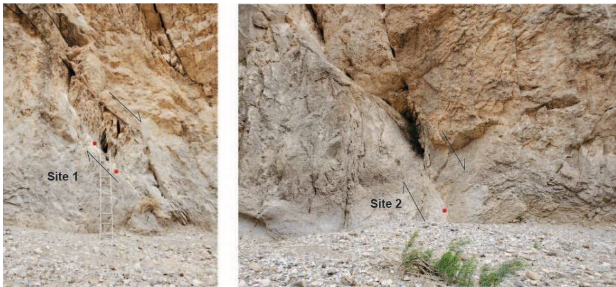
Figure 3.19. Two pull-apart structures on Dog Canyon's south wall at the canyon floor with annotated senses of motion (arrows) and locations of measured slickenlines (red squares). Site 1 is west of Site 2. Ladder for scale in left image; right image is of similar scale.
