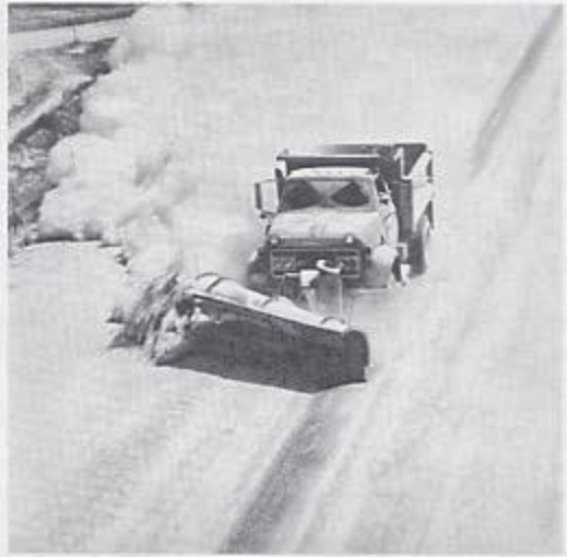
Figure 412.—Removal of ash from the May 18 eruption, Interstate 90, eastern Washington. Photograph by Washington State Highway Department.
