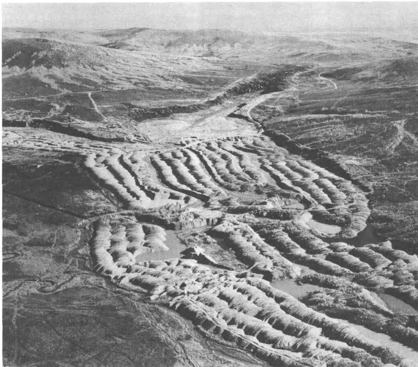
FIGURE 2.—Low oblique air view looking southeast near junction of Engineer and Goldstream Creeks, Fairbanks. Gravel dredge tailings in foreground and to left are on Goldstream Creek. Frozen silt removed from creek-valley bottom by hydraulic stripping is exhibited on Engineer Creek in middle ground. (Photograph 2414 by Bradford Washburn, September 1936.)
