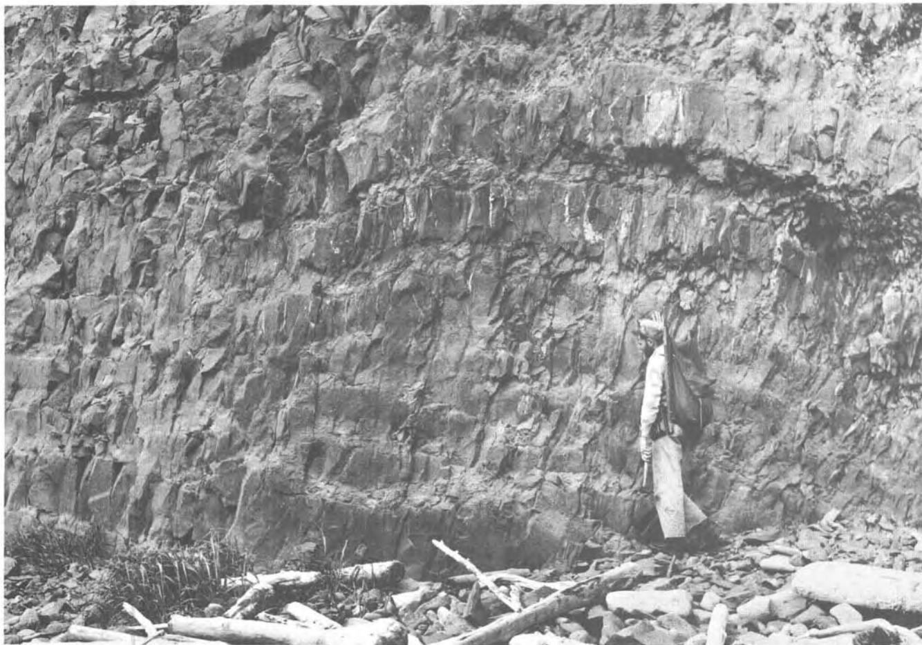
FIGURE 12.—Layered albitized dacite lava pod in active sea cliff west of Buttress Point, Unalaska Island. Closeup of central part of Figure 11. Specimens for chemical analyses 2, 3, and 5, table 2, were collected from the resistant and nonresistant layers just over the geologist's head. Resistant layers contain quartz, and nonresistant layers contain a carbonate.
