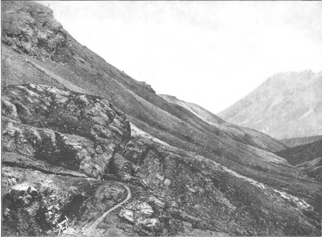
4. VIEW OF NIKOLAI MINE ACROSS UPPER NIKOLAI CREEK.
