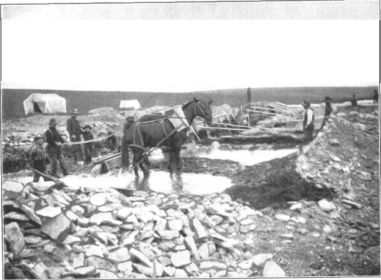
A. SLUICING ON INMACHUK RIVER
